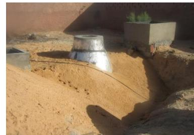
Construction of the gasometer tank the diameter of the first circle is 300 cm, the second having a diameter of 250 cm.
