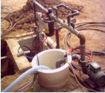
Fig. 3: Feed pump
